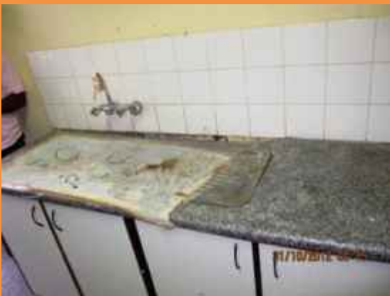
A broken sink
